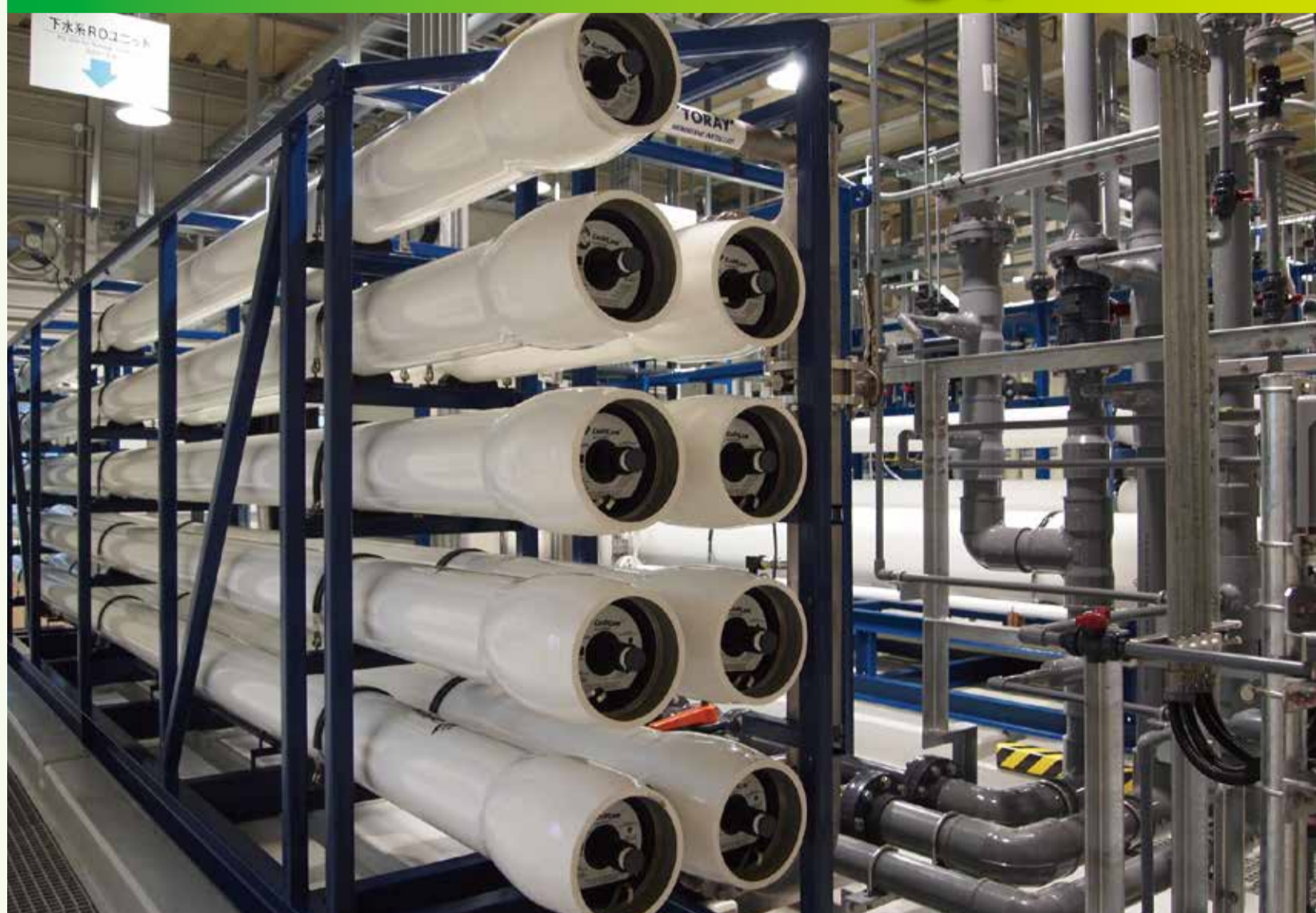
Arrangement of site visits to wastewater treatment plants
